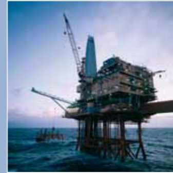
Water intake – seawater, brackish water, surface water
